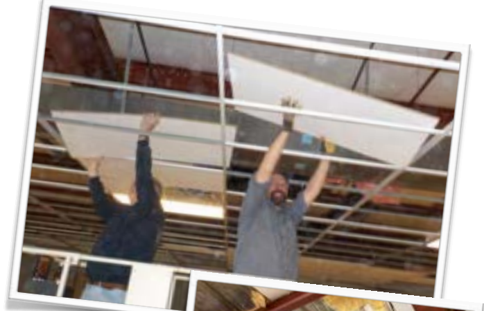
Ceiling work begins as old tiles come down, insulation is removed, and spray paint begins.
