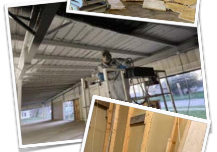
Openings will be cut for the new layout.
