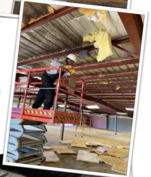
Ceiling work begins as old tiles come down, insulation is removed, and spray paint begins.
